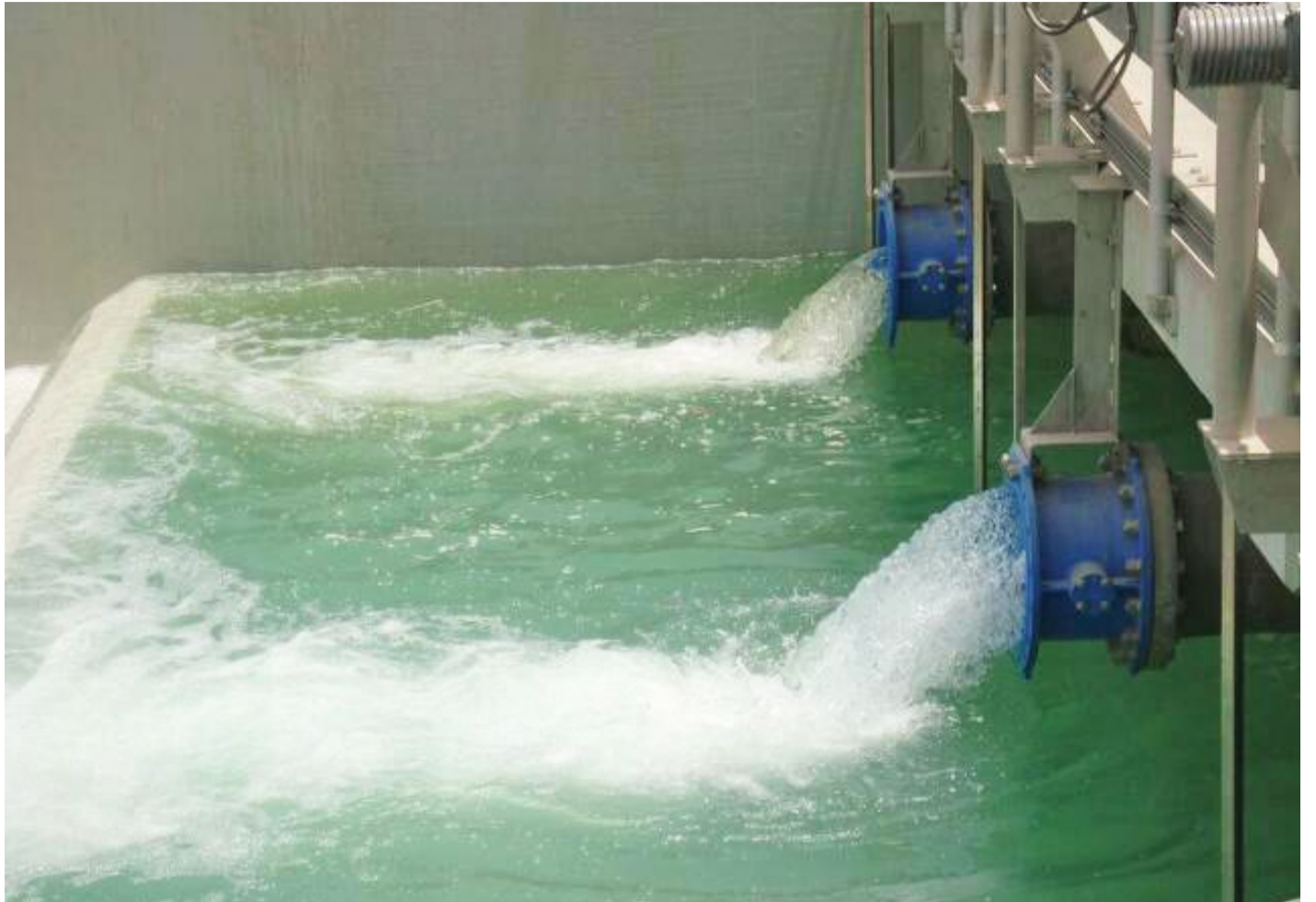
Seven hundred farms directly benefit from the Tubli Wastewater Treatment Plant.
